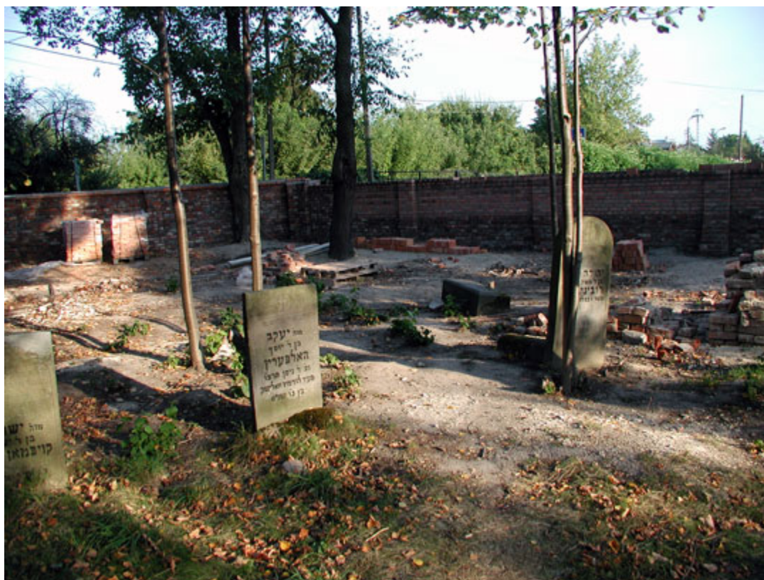
Completed segment of wall repaired in August 2008.
