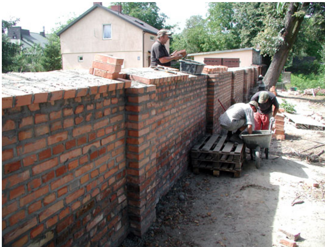
Finishing of the segment of wall repaired in August 2008.
