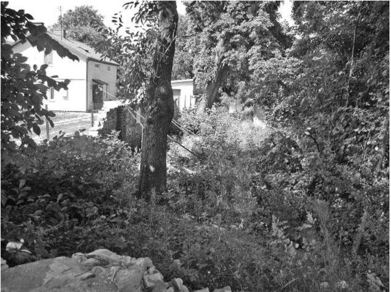
Condition of wall June 2008.
