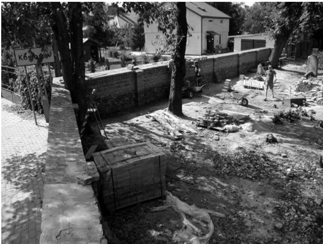
Completed segment of wall repaired in August 2008.
