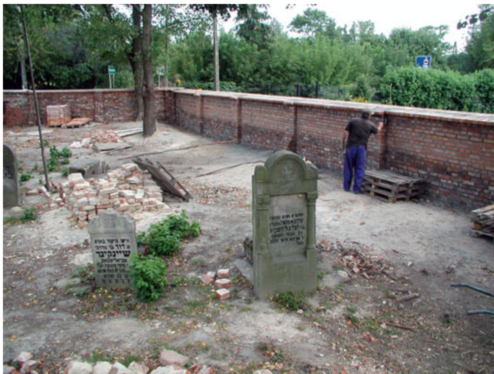
Completed segment of wall repaired in August 2008.
