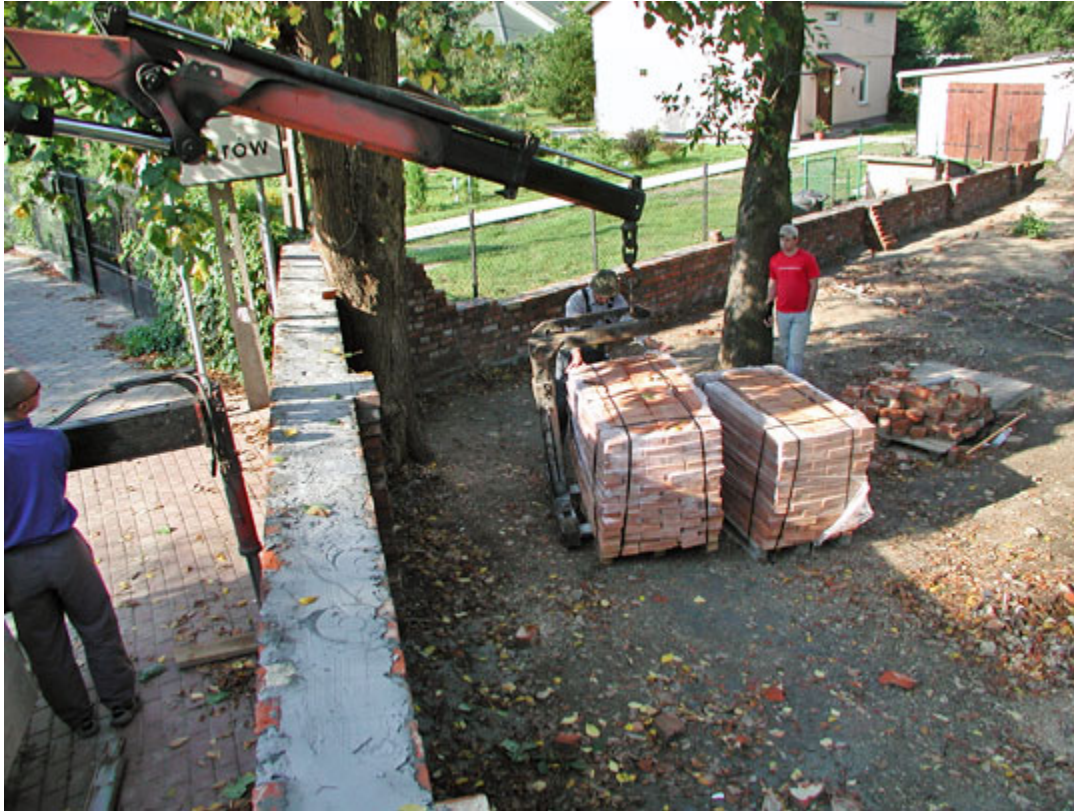
Final stage of completing the restoration of the wall segment at Pruszkow (August 2008).
